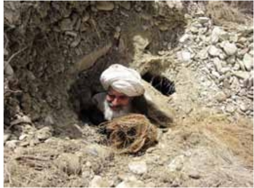
Figure 20. A specialized Karez cleaner in Qila Iskan Khan, seen with a dot of grass removed from the underground canal bed. Due to the high risks involved and the special skills required, it is a well-paid job (Photo: IUCN Pakistan, 2010).
