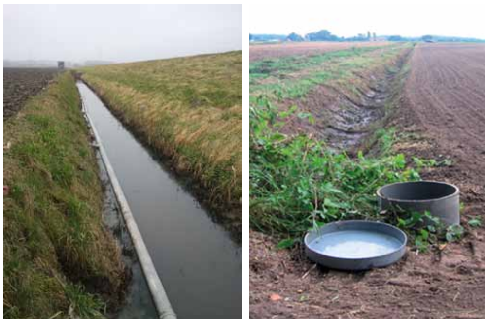
Figure 32. a) Controlled drainage installed in fields in the Netherlands, where the drains are connected to a collector drain; b) and a vertical pipe which acts as the control unit for the water level. (Photos: Acacia Water)
