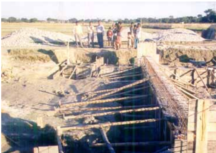
Figure 34. Constructing a gully plug to retain groundwater (Photo: Richard Soppe)
