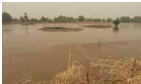
Figure 45. ‘Hout’ infiltration pond in desert area of Kassala (Sudan): this is an example of A2. The desert village of Weger depends on entirely on wells fed from the infiltration pond that is recharged annually with flood water from the Gash river). The wells are seen in the middle of the pond (Photo: Abraham Mehari Haile).
