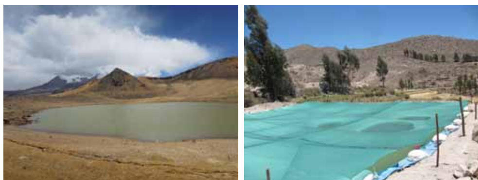
Figure 42. a) High altitude storage pond; b) Covered open water basins to buffer spring water (Photos: Acacia Water).
