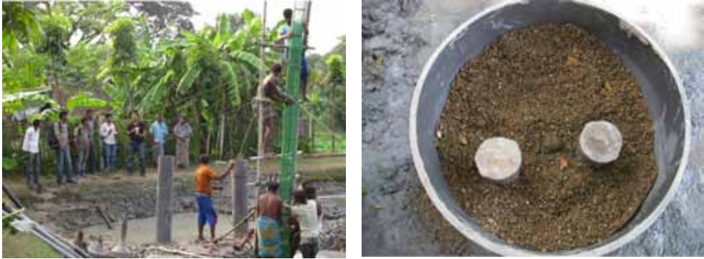
Figure 29. a) Well construction; b) Typical infiltration well
