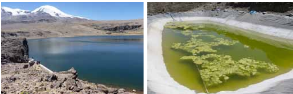
Figure 10. Open water storage behind a check dam (a) and in a plastic lined pond (b) in the Andes, Peru (Photo: Acacia Water).
