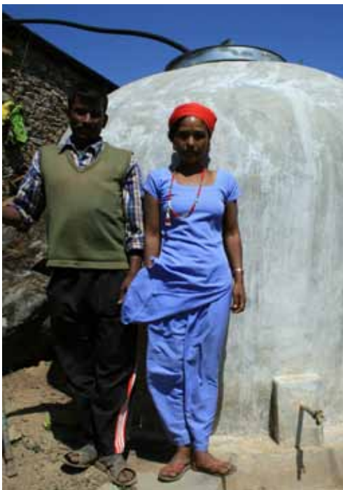
Figure 44. Rainwater storage, Nepal. (Photo: Acacia Water)
