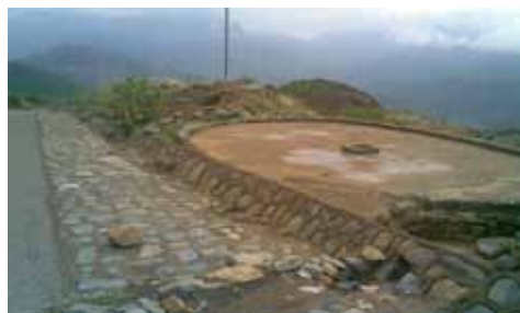
Figure 46. Collecting road runoff in a cistern (Yemen) - the first flush is left out as it is contaminated (Photo: Mohammed Al Abayad)
