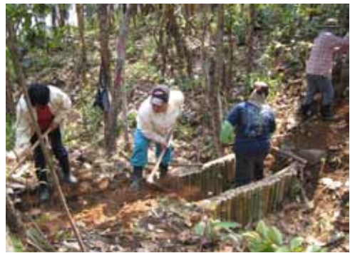
Figure 18 a and b. Villagers were building a basic check dam across one of the small gullies with local materials. (Photo: Hydro and Agro Informatics Institute (HAI), Bangkok)
