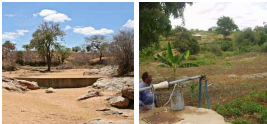
Figure 15. a) Sand storage dam; b) Fetching water in Kitui (Photo: Acacia Water).
