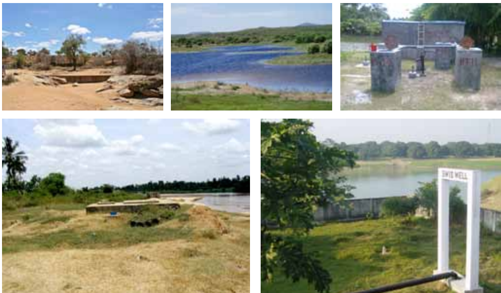
Figure 6 a, b, c., d, e. Different types of recharge (Photos: Acacia Water).
