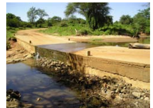
Figure 3: Irish bridge (Source: Nissen-Petersen, E, 2006)
