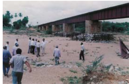
Figure 3: Railway bridge foundation frequently being repaired due to sand mining across Uttara Pinakini river in Gauribidanur taluk, Karnataka, 2002. (Hemalatha, A.C. et al. 2005)
