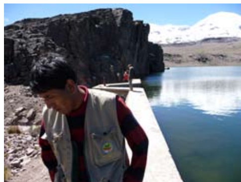
Figure 1: A retention dam at Lago Palcacocha, near the Coropuna Glacier
