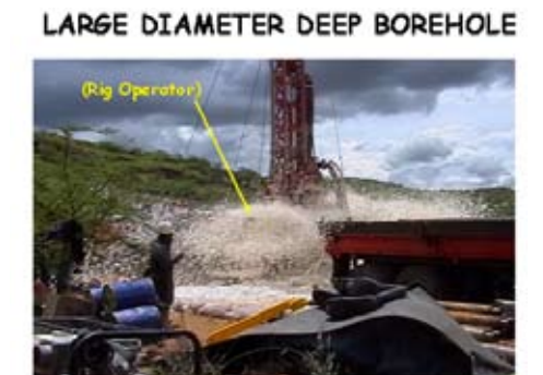
Figure 4: Drilling of large diameter deep borehole
