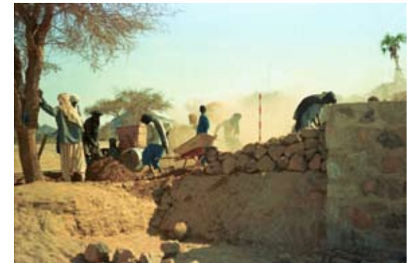
Figure 2: Construction of diversion works
