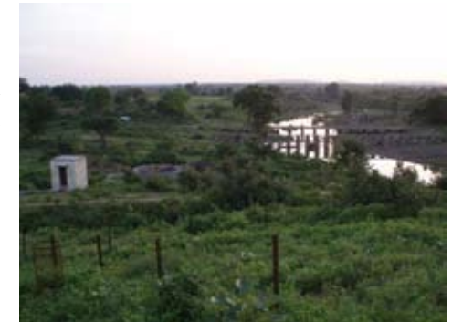
Figure 2: River bank infiltration well in Maharashtra
