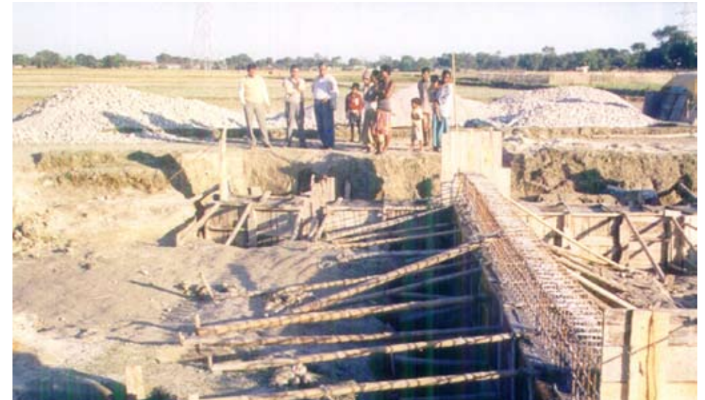
Figure 2: Constructing a gully plug to retain groundwater
