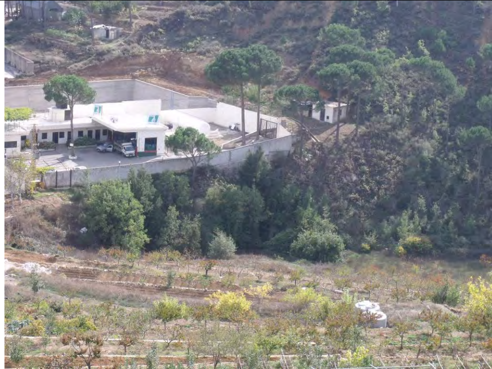
Sinkhole next to gas filling station
