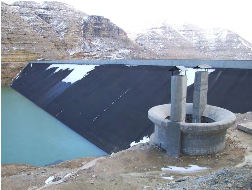
Figure 81: Chabrouh Dam with Overflow Structure in February 2011
