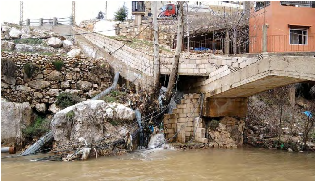
Figure 126: Sewage canal discharging into Nahr el Salib at Hrajel
