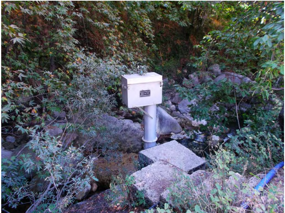
Figure 27: Rouaiss spring discharge monitoring station 222
