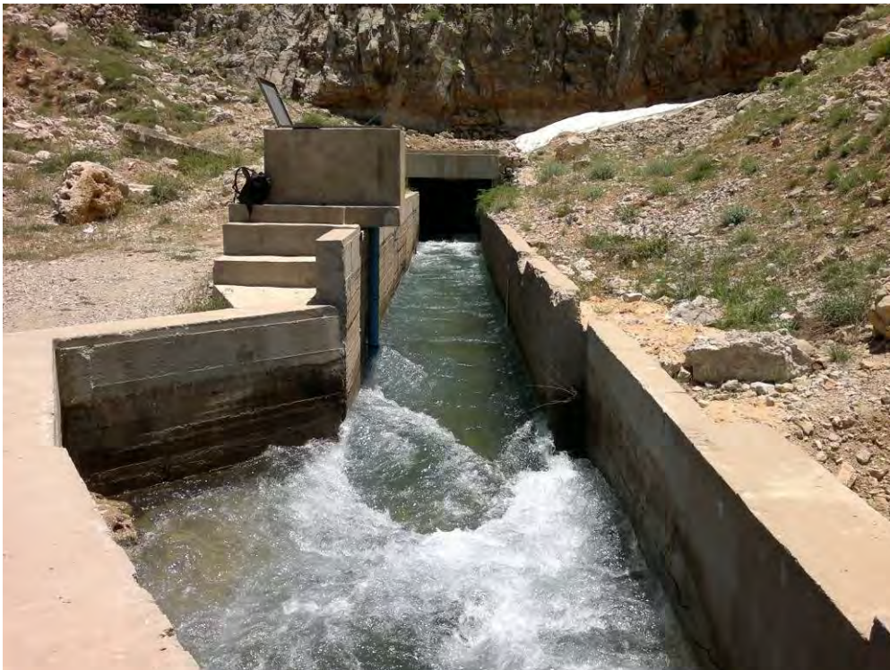
Figure 62: Labbane spring with multiparameter probe (in blue PVC casing) protected by a locked concrete box
