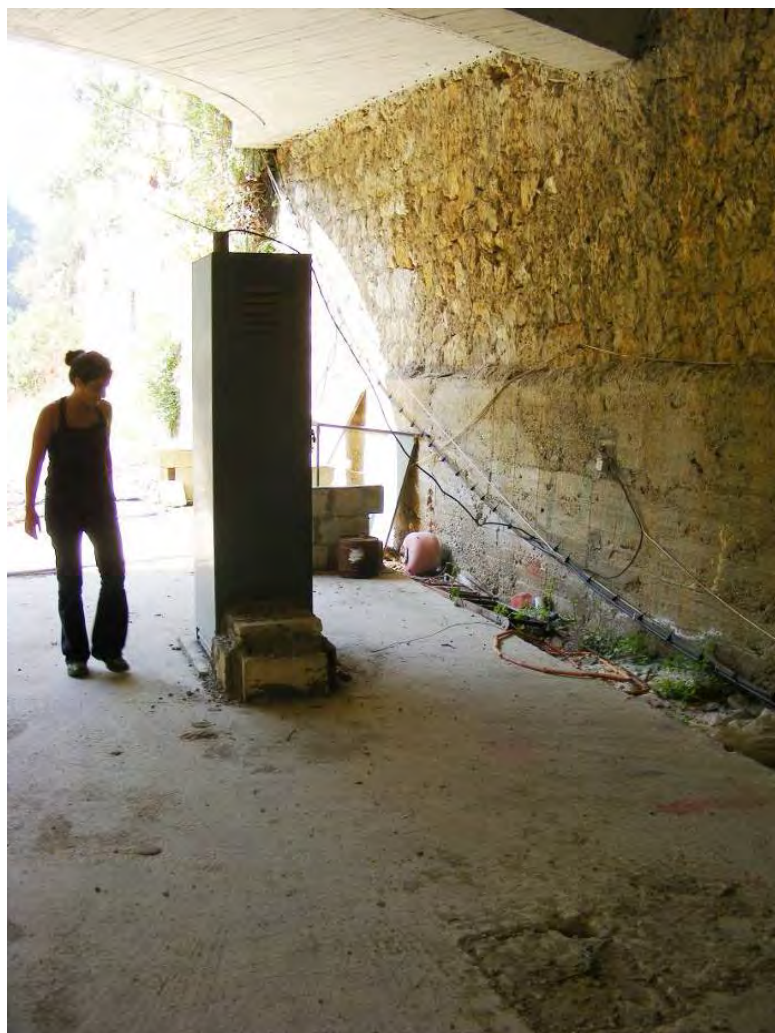
Figure 20: LRA Discharge Monitoring Station at MAPAS parking
