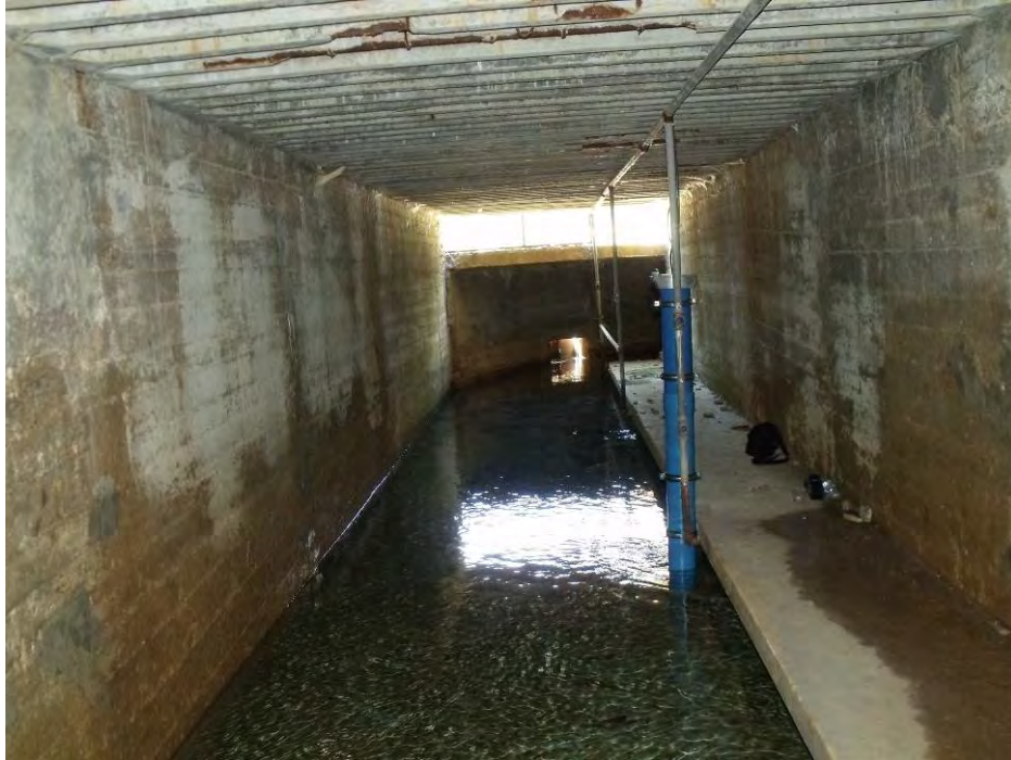
Figure 55: Multiparameter probe Troll 9500 installed in Assal spring
