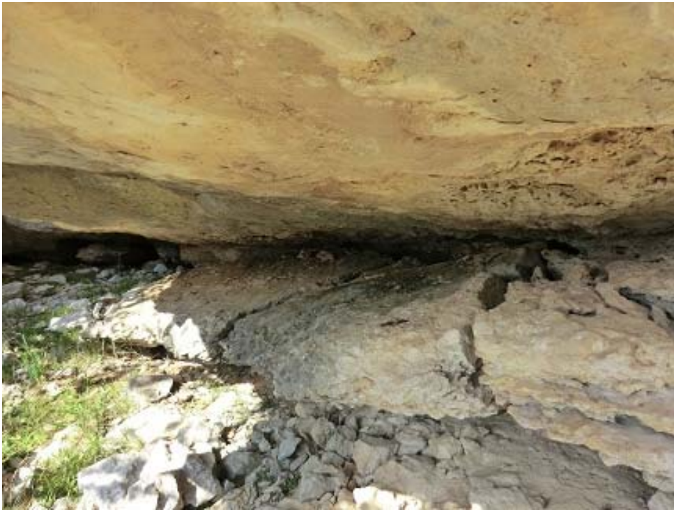
Figure 31: Erosion Progressing along Soft Rock Layer at Bedding Plane (WP67)
