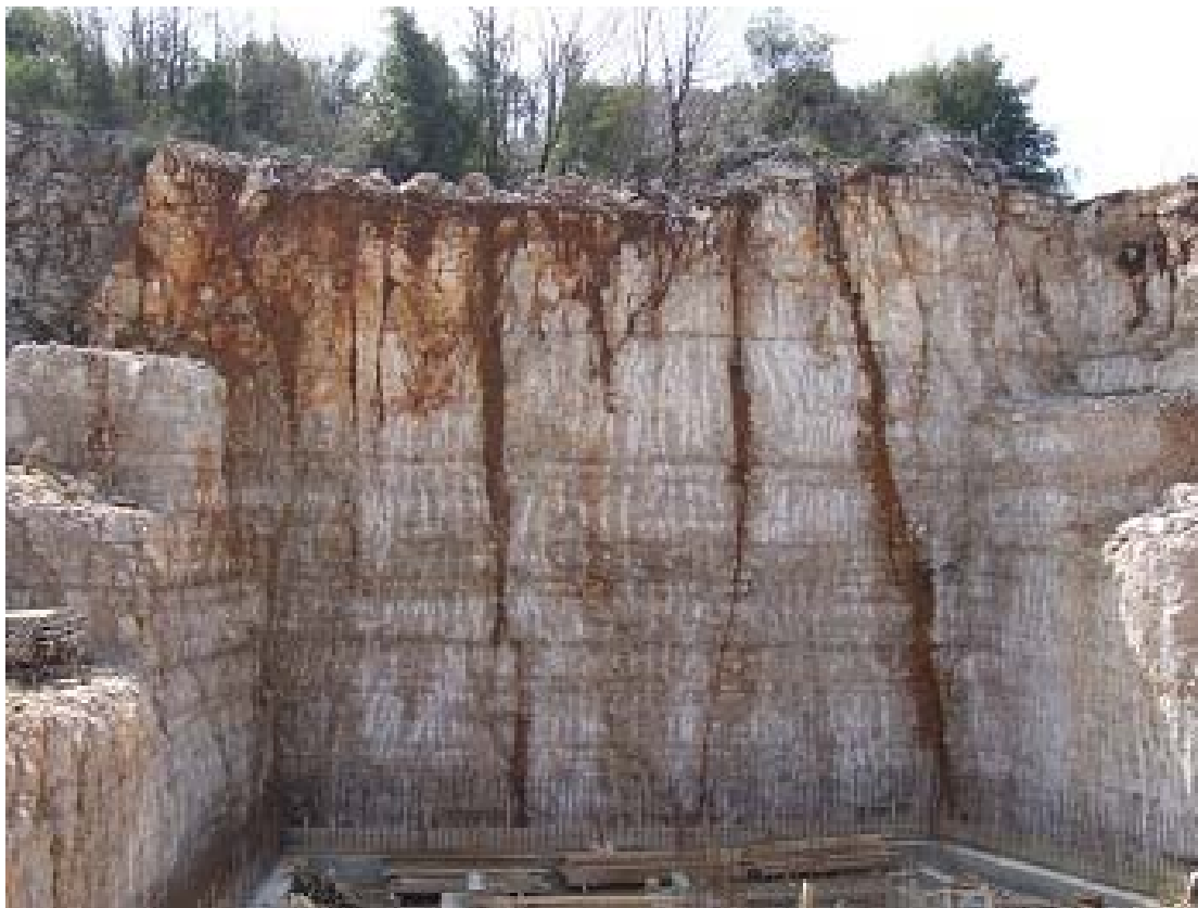
Figure 45: Fissures filled with Soil without Indication at the Land Surface (WP53)
