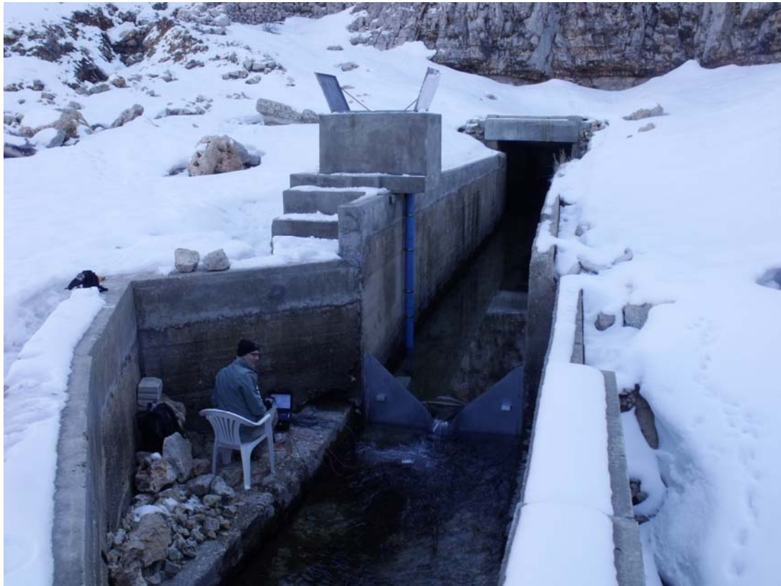
Figure 12: Weir at Labbane Spring and Multiparameter Probe installed in a Casing with Telemetric Data Transfer
