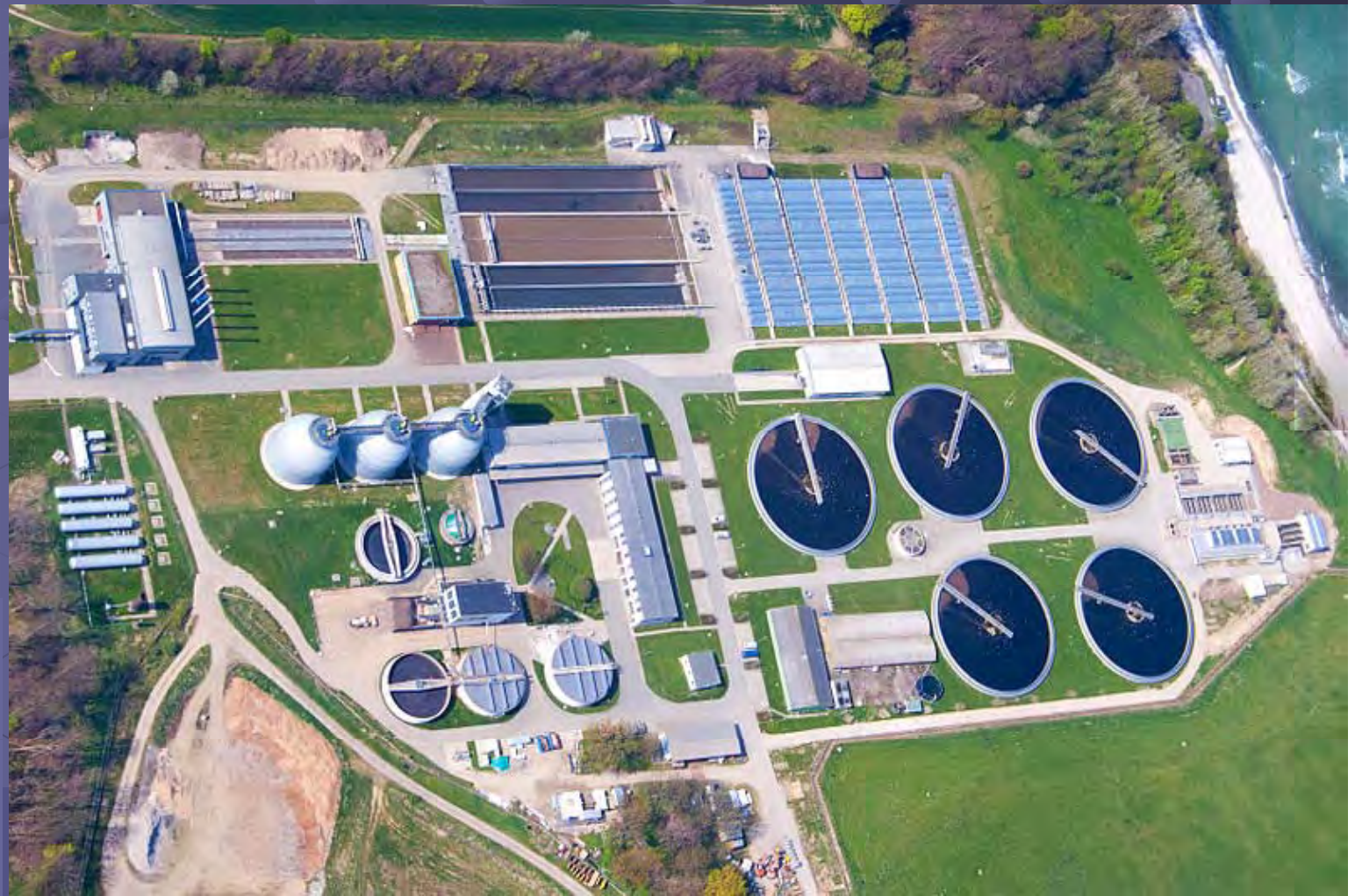
Wastewater treatment Plant (WWTP) Kiel/Germany 380,000 PE (PE-person equivalent)
