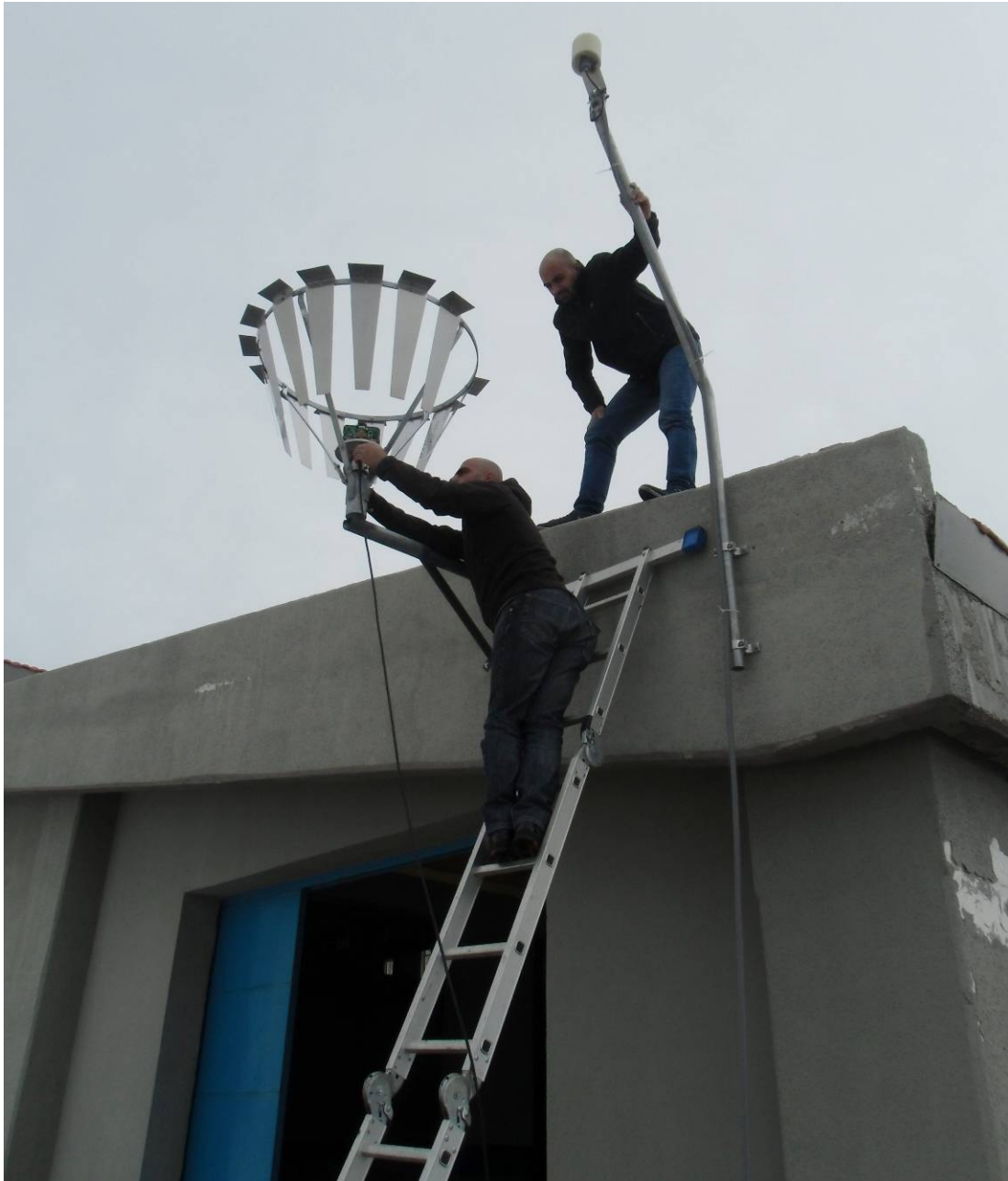
Figure 11: Installing a Weather Station
