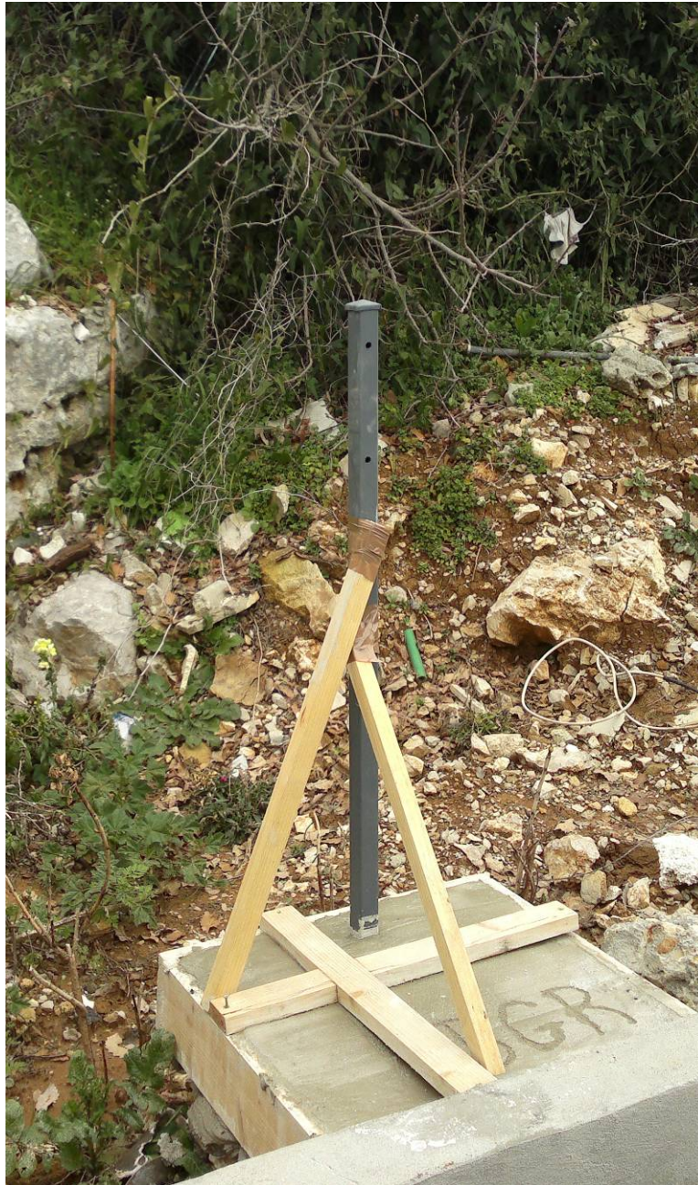
Figure 16: Making the Concrete Base
