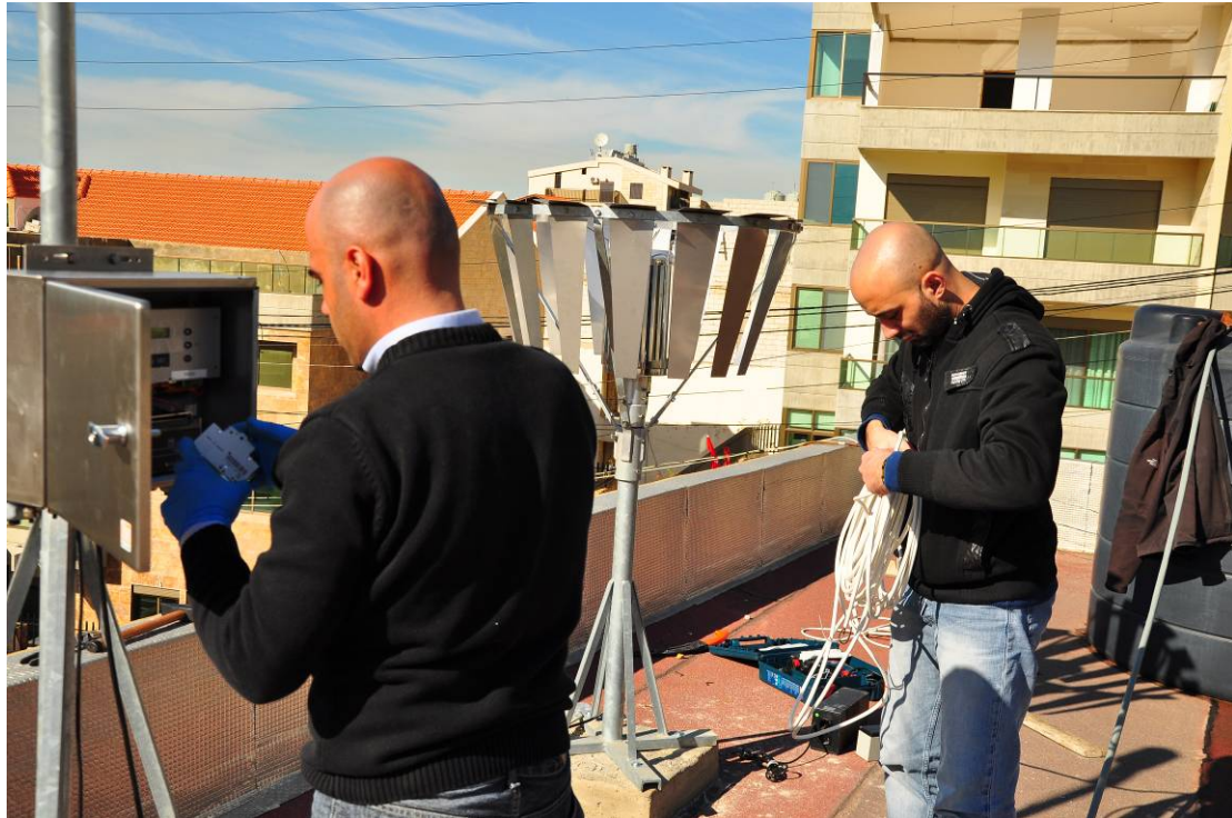
Figure 12: Installing the individual Components of a Weather Station
