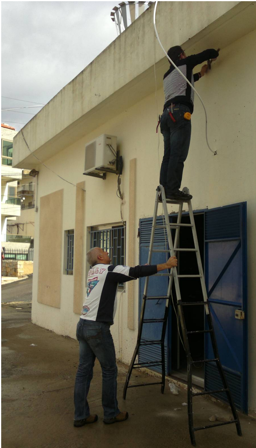
Figure 13: Installing the Power Supply to the Station
