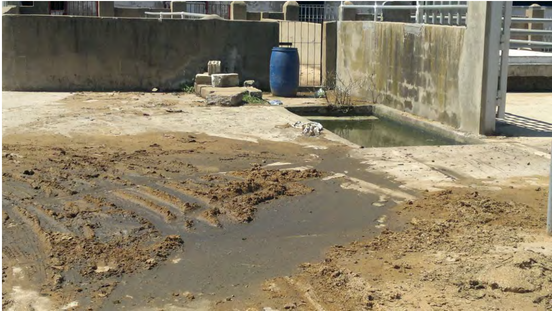
Figure 55: Basin filled with insecticide, once fully used the rest will be discharged without treatment in the above mentioned cesspit at Ghosta slaughterhouse
