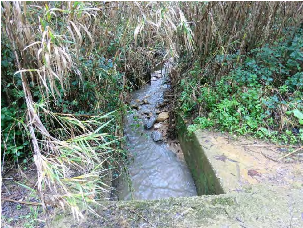
Figure 27: Wastewater discharge into Nahr el Kalb at Jeita
