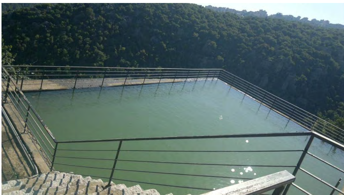
Figure 89: Water reservoir collecting the used water for further reuse
