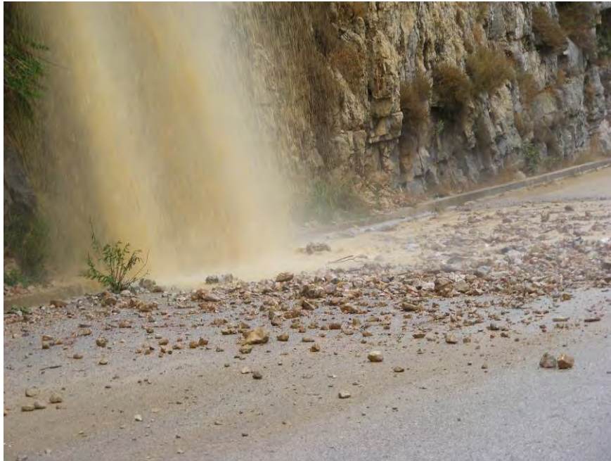
Figure 45: Stormwater carrying stones and soil damaging the road in Bquaatouta during a rainy day
