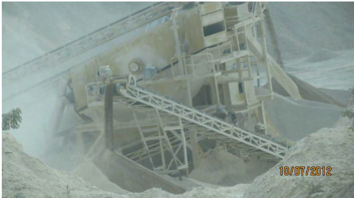
Figure 62: Dust generated during aggregates processing at Mehanna quarry, Wata el Jaouz
