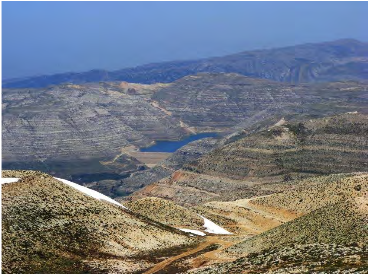
Figure 11: View of Chabrouh Dam from Mzaar
