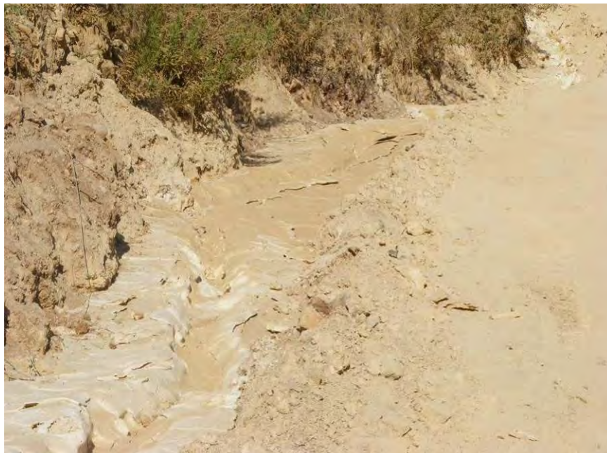
Figure 44: Gypsum Sludge resulting from quarries and cutting blocks disposed in the storm water canal on a road side
