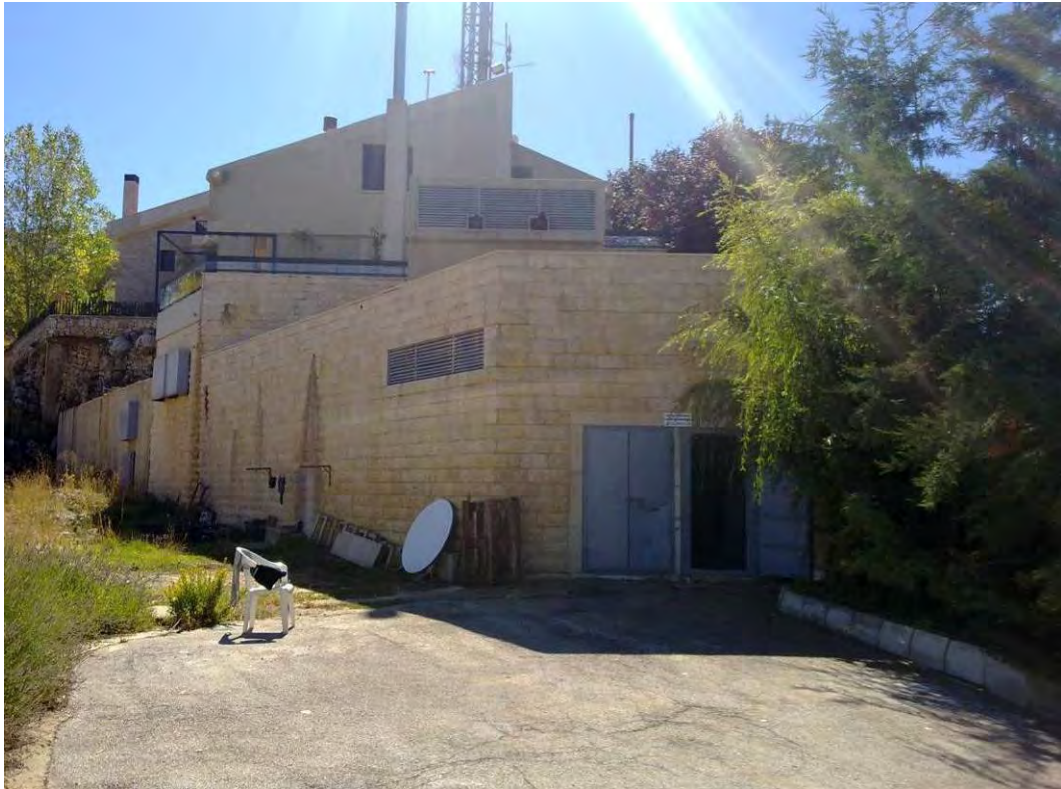
Figure 23: Wastewater Treatment Plant of Faqra Club
