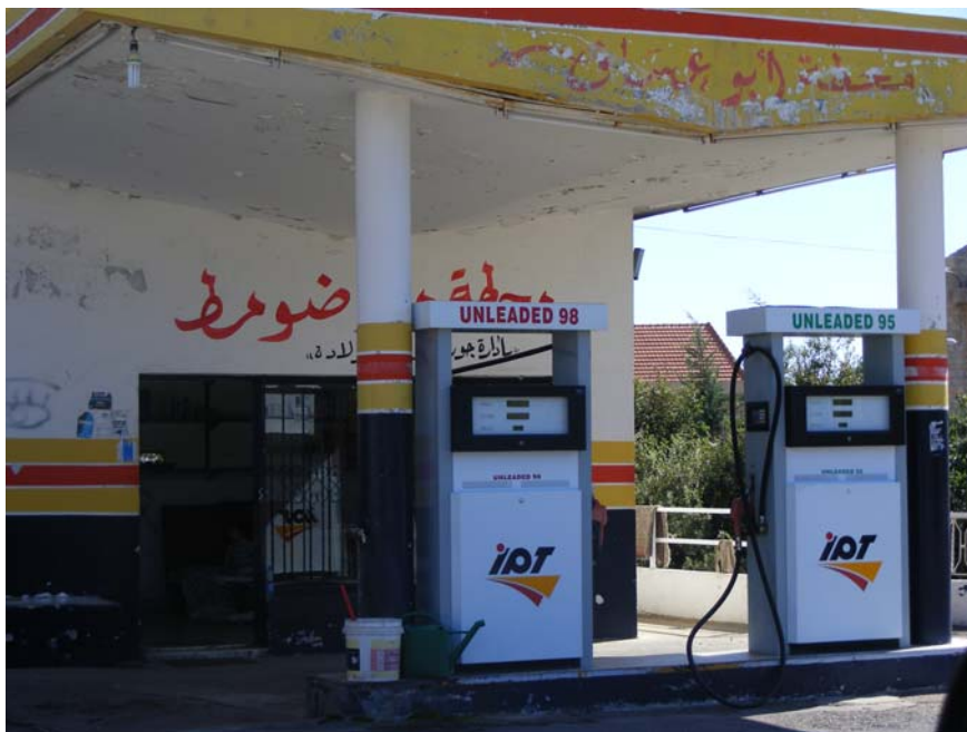
Photo 4: Gas station selling fuel 95 and 98 octane including only one fuel storage reservoir
