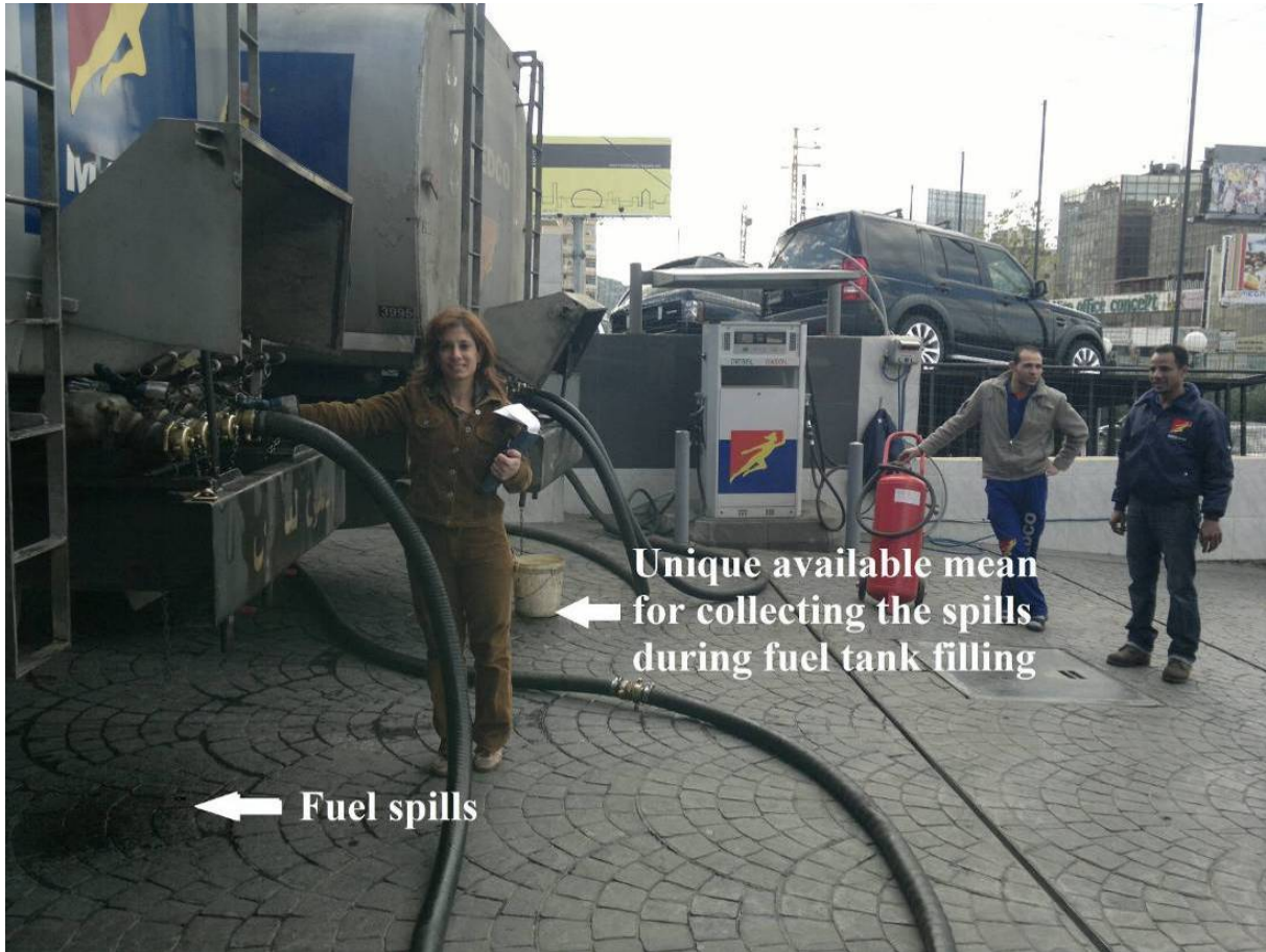
Figure 28: Spills while filling underground fuel tanks
