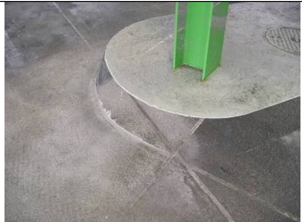
Sealed joints in good conditions
