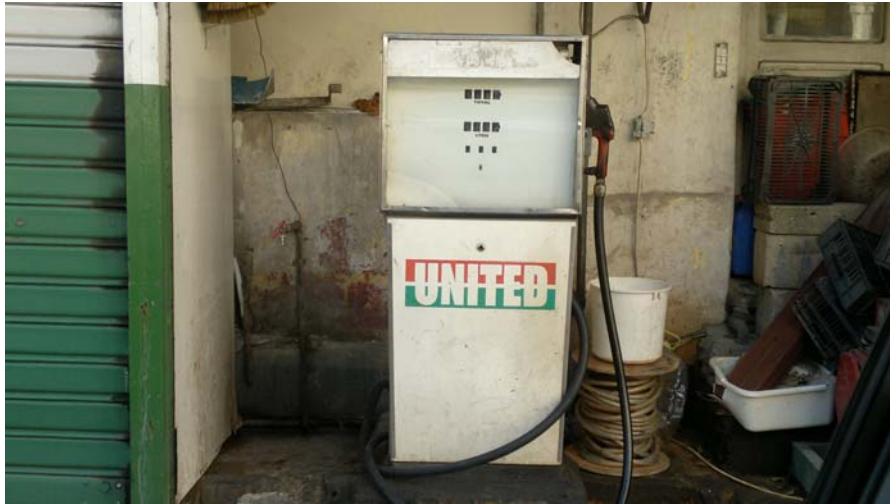
Photo 3: No umbrella to protect diesel oil distributors from rainfall waters...
