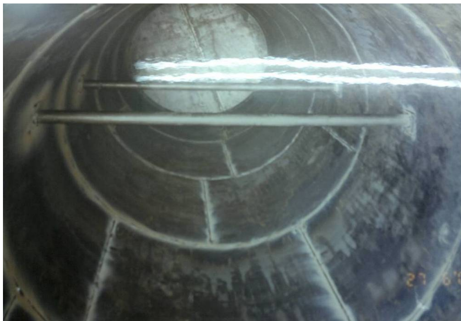
Figure 18: Internal shape of a tank shot taken during the welding process
