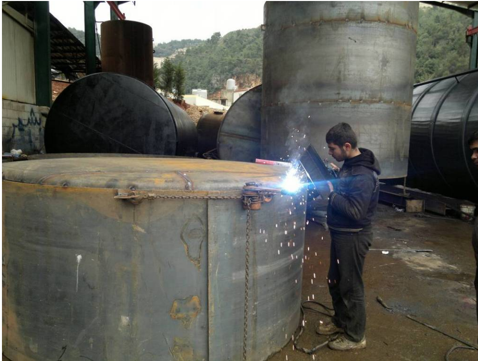
Figure 17: Joining the tank concave extremity by welding.
