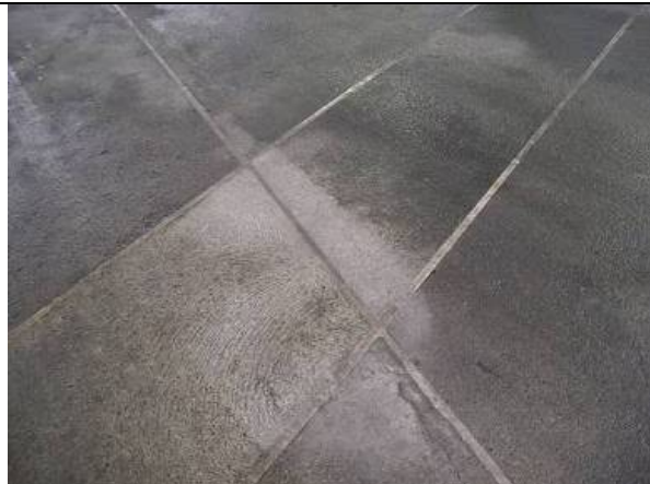
Sealed joints in good conditions
