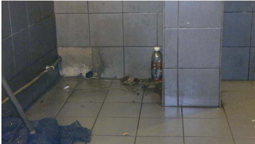
Photo 10: Hole in the wall leading to a leaking cesspit used to evacuate lube change cleaning effluents at a gas station located in the Jeita groundwater Catchment, and piece of cloth contaminated by oil spills.
