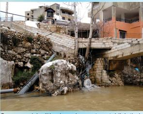
Some municipalities have begun to establish their own WW networks. However, these are mostly poorly constructed and discharge untreated WW into the rivers. They can not be used by the new WW projects.
