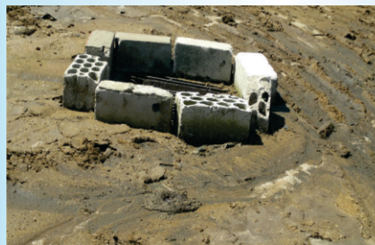
Liquid waste disposal: effluent is discharged into a borehole without treatment, in absence of a proper drainage system.
