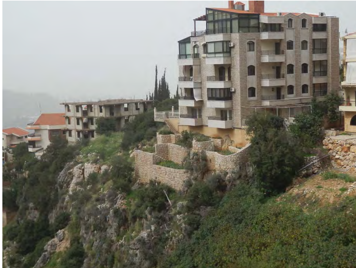
Figure 9: Wastewater discharge into valley from residential buildings
