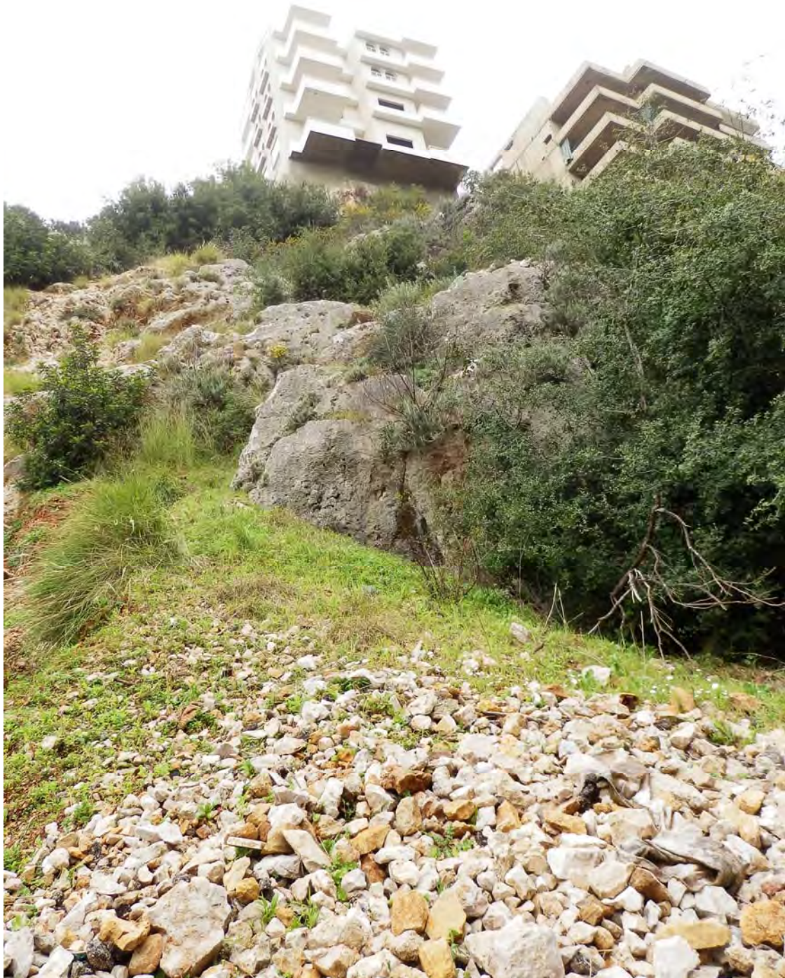
Figure 7: Construction of multi-storey buildings at the escarpment of the valley with dumping of construction waste into the valley
