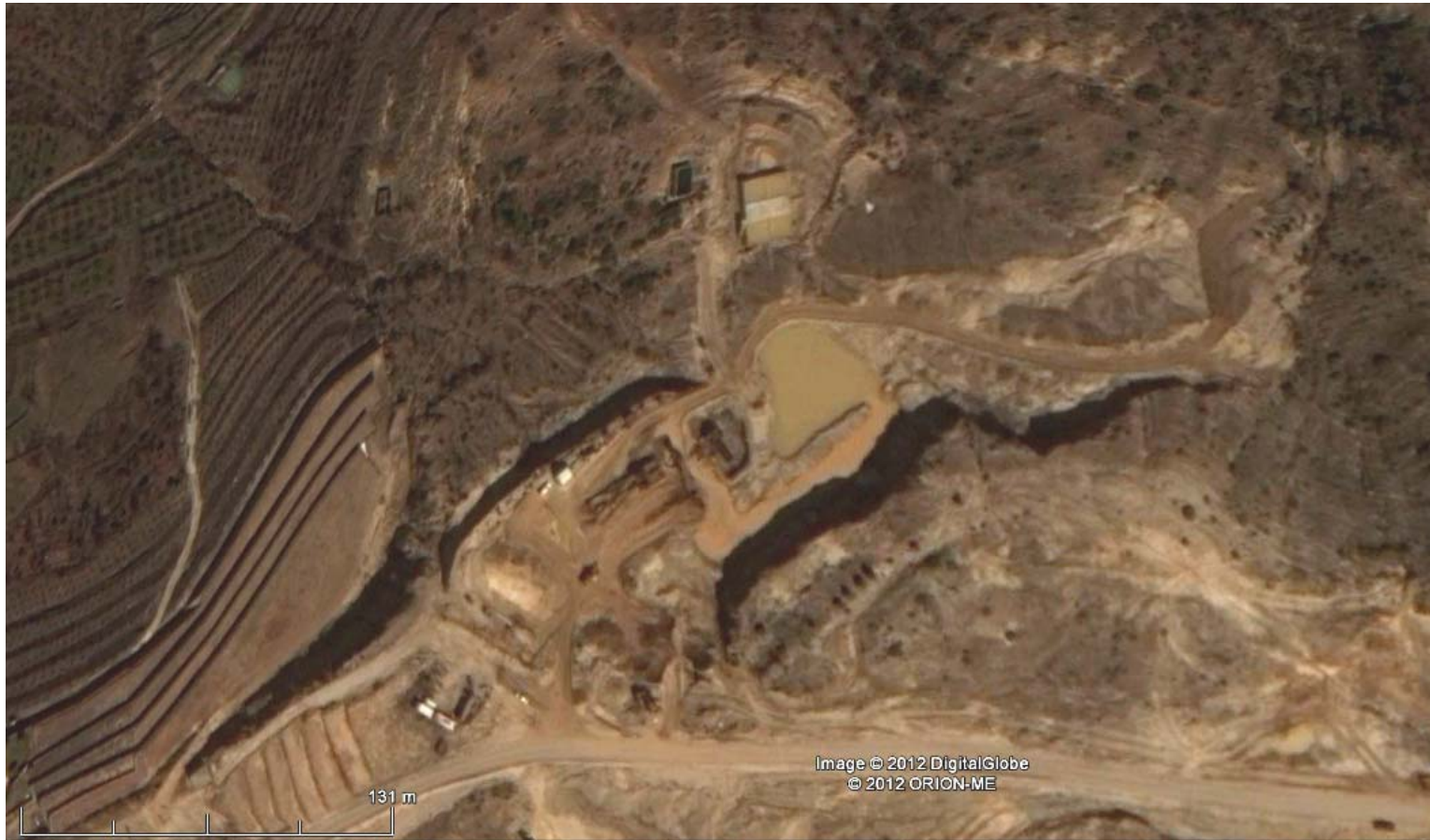
Figure 41: Water Pond used for Sand Washing and Flushing of Fine Material in Sandstone Quarry of HAJJ Contractors/Bqaatouta
