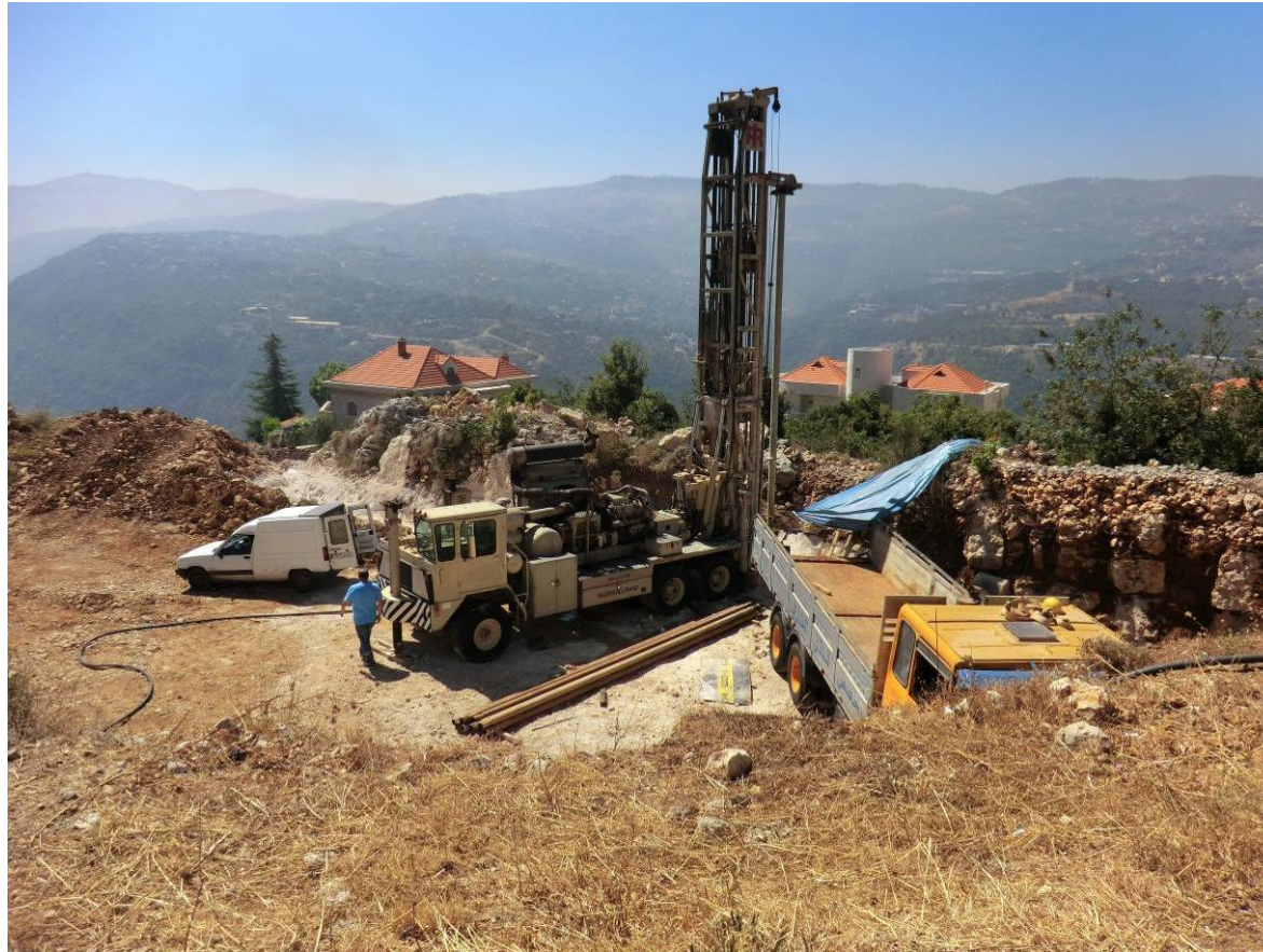
Figure 14: Drilling of Joseph Nassar Water Well in Ballouneh
