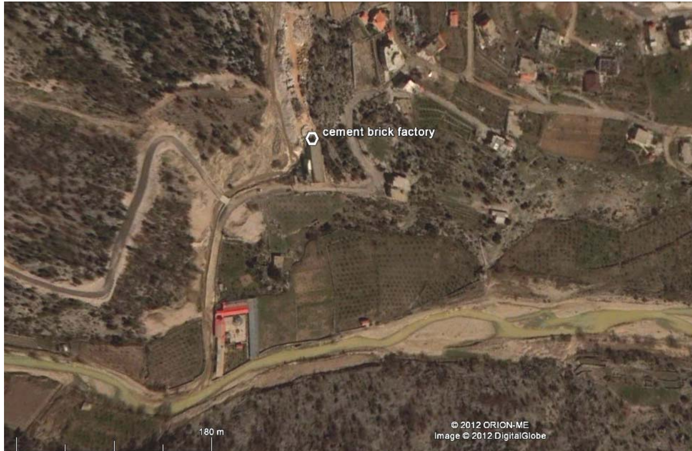
Figure 29: Cement Brick Factory in the Upper Nahr es Salib at Mayrouba
