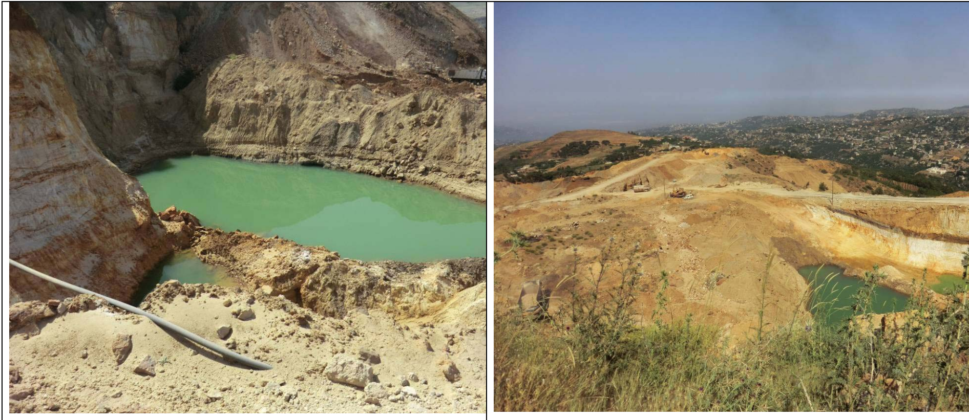
Figure 38: Water Ponds in Sandstone Quarry of HAJJ Contractors in Bqaatouta
