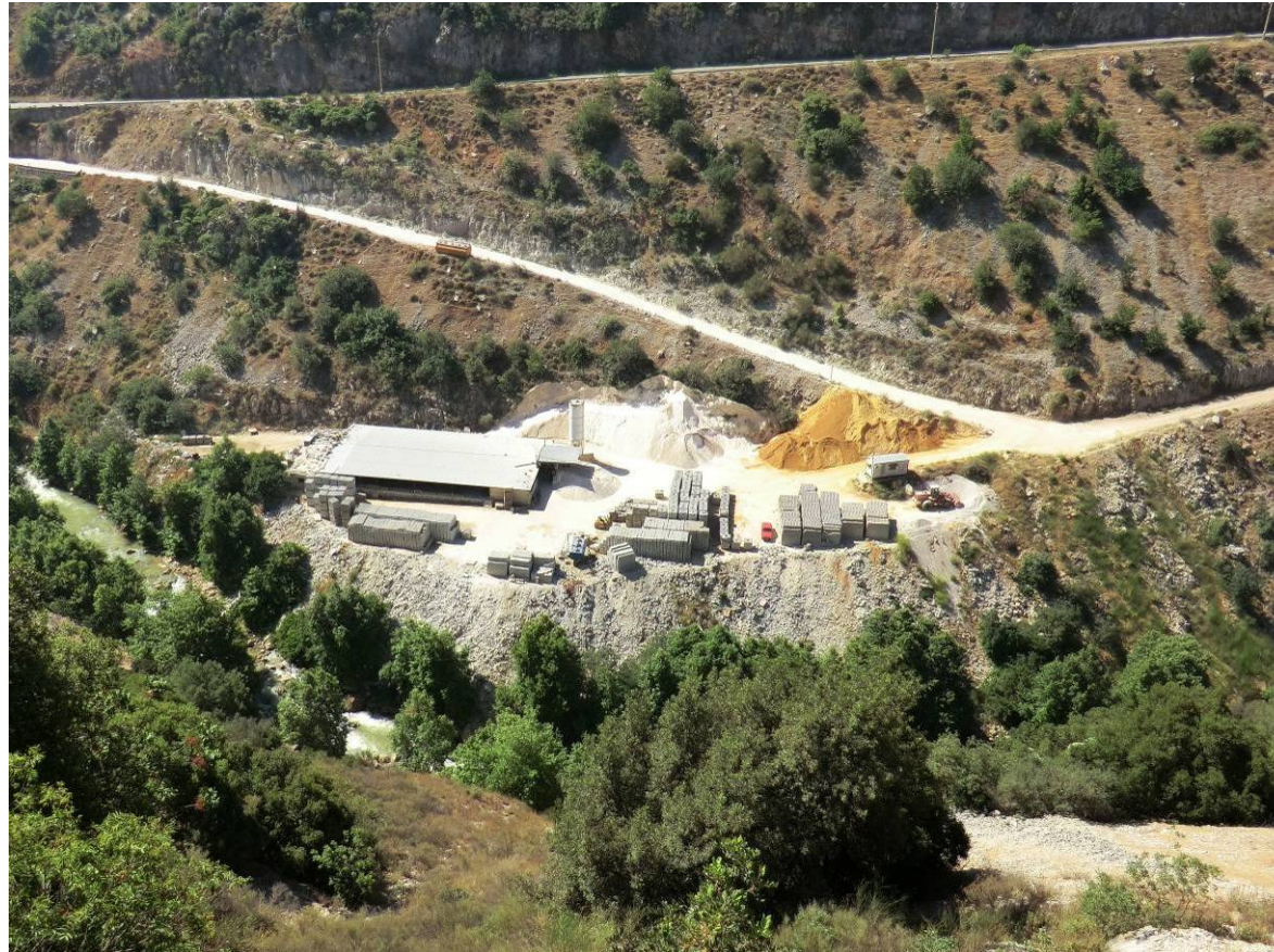
Figure 18: Cement Brick Factory in Lower Nahr es Salib
